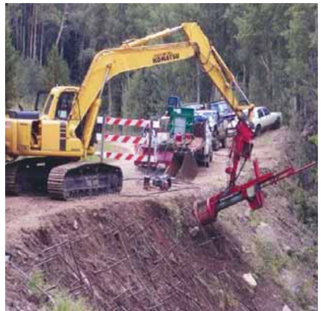
Figure 3 - Typical Launched Soil Nail Slope Repair
