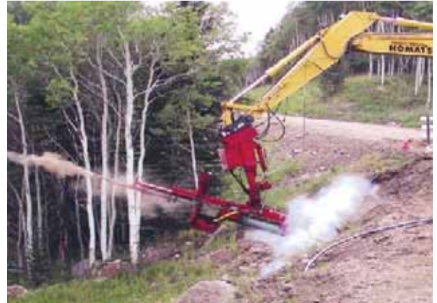
Figure 2 - Soil Nail Launcher in Action
