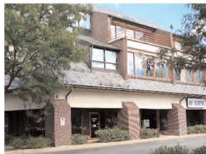
ARM State College office building
